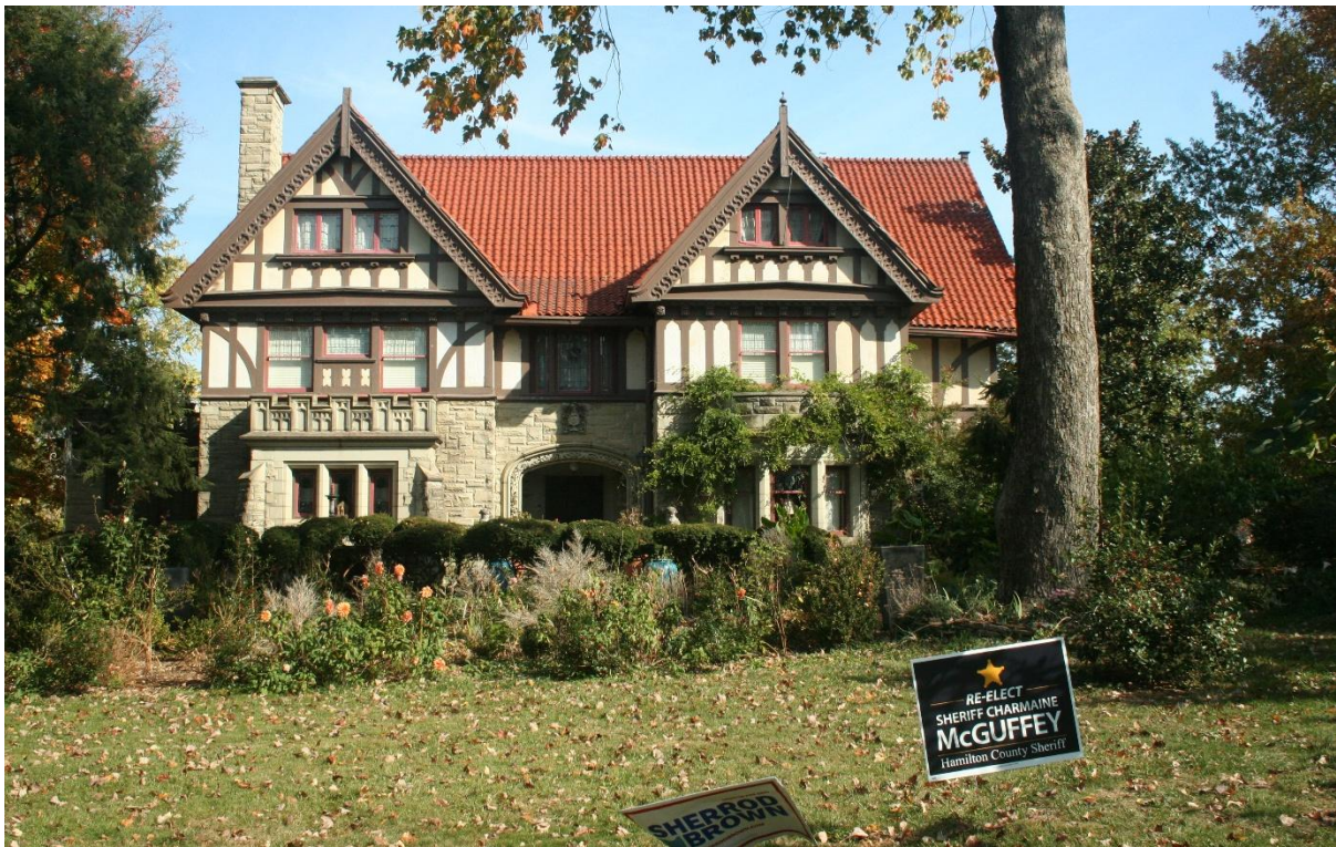
Photo 1. 4008 Rose Hill Avenue (1980), C. M. H. Atkins House, John Scudder Adkins, Tudor Revival.
