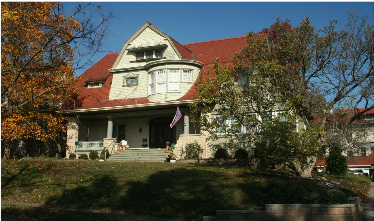
Photo 17. 1006 Lenox Place (1900), Shingle style.
