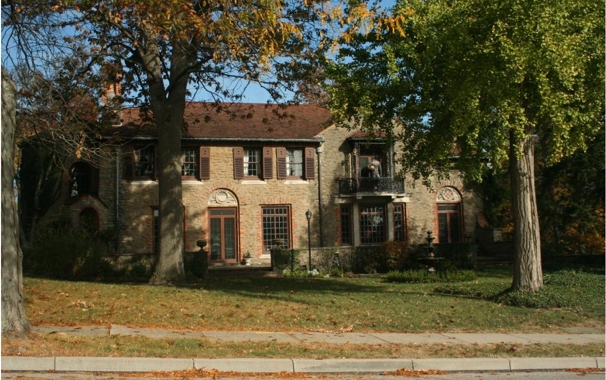
Photo 2. 960 Avondale Avenue (1912), Harry L. Linch House, Grosvenor Atterbury, Italian Renaissance.
